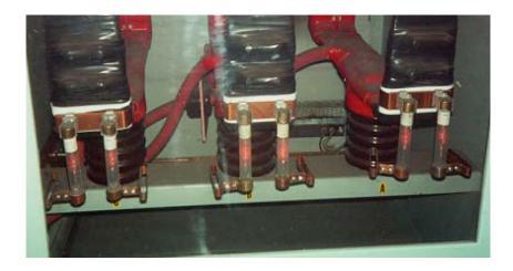
WARNING: GLOW TUBES CAN NEVER BE USED AS A SOLE DEVICE TO CONFIRM VOLTAGE PRESENCE. OTHER DEVICES ARE NEEDED TO VERIFY PRESENCE OF THE VOLTAGE ON THE BUSBARS/CABLES. BUS BARS MAY NOT BE DEAD IF GLOW TUBES ARE NOT LIT!
